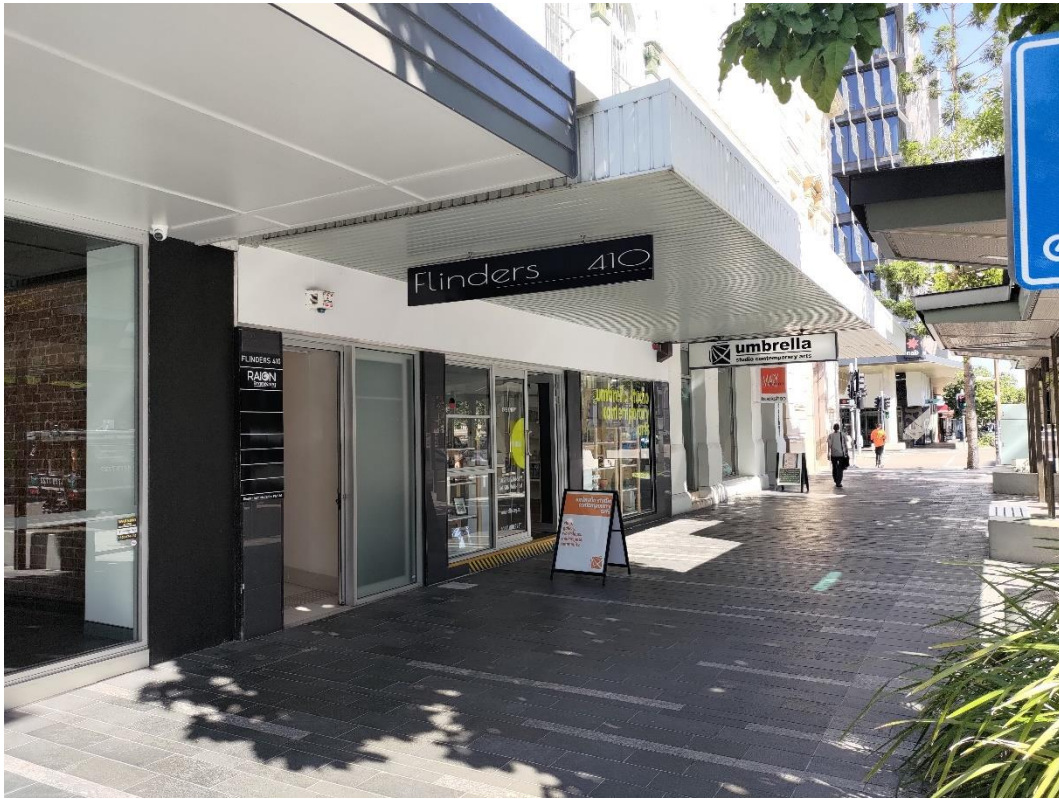
Figure 5: Flinders Street frontage, ground floor (Queensland Government, 2023)
