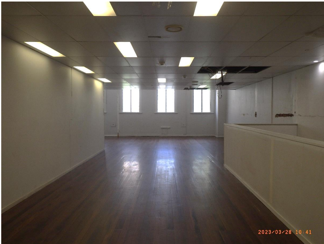
Figure 9: First floor, 1902 section, looking to front wall (Queensland Government 2023)
