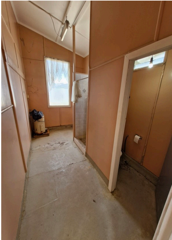
Figure 10: Bathroom in office block of Base Building (Queensland Government, 2024)
