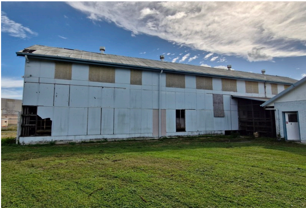
Figure 6: Southern side of Base Building (Queensland Government, 2024)
