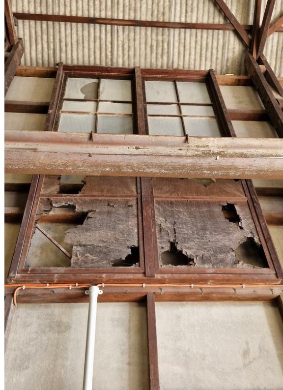
Figure 8: Original fixed window with blackout sash (Queensland Government, 2024)
