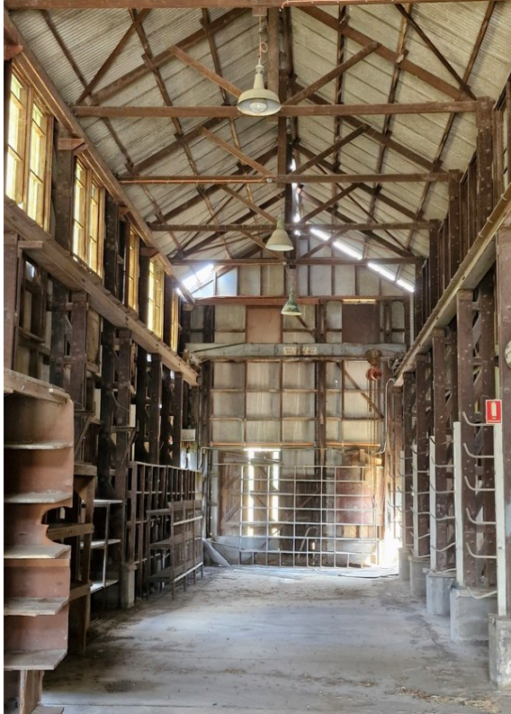
Figure 7: Interior of Base Building looking west (Queensland Government, 2024)
