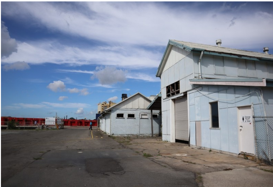
Figure 4: Base Building, eastern end with wharf in far background (Queensland Government, 2024)
