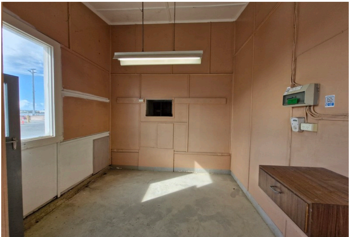
Figure 12: Former office in office block of Base Building (Queensland Government, 2024)
