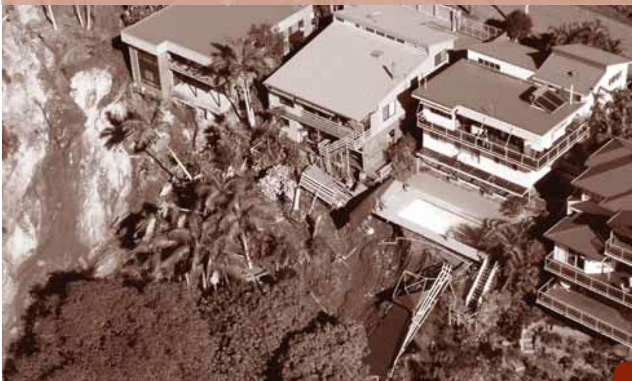
Landslide at Currumbin June, 2005.
