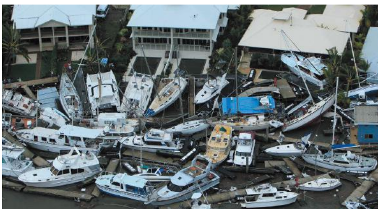
Figure 36: The aftermath of Cyclone Yasi as it crossed the Far North Queensland coast. Dozens of luxury boats were smashed together at the Port Hinchinbrook marina in Cardwell. Source: Marc McCormack
