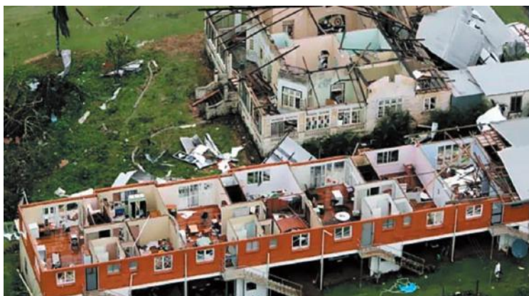
Figure 34: Houses and apartment blocks with their roofs blown off in Innisfail after Cyclone Larry struck in March 2006. Source: Mark Baker(AP)
