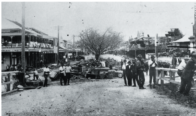
Figure 30: Looking south down Sydney Street post the impact of the 1918 Mackay Cyclone.
