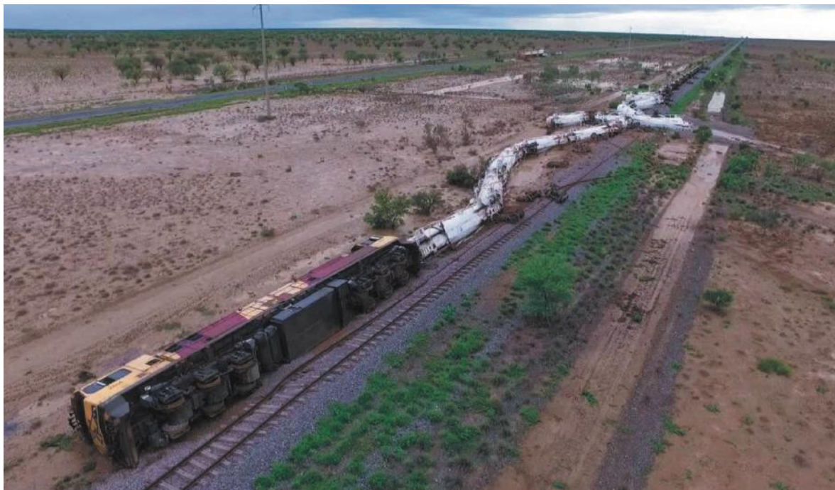
Figure 98: Derailment of freight train near Julia Creek, 27 December 2015. Source: Queensland Police Service.
