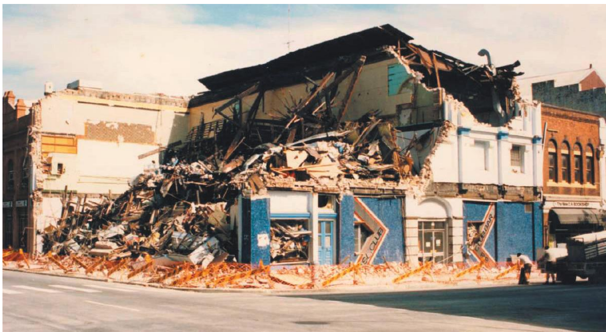
Figure 84: Damaged caused by the 1989 Newcastle earthquake was significant and destructive. In this photo, the RSL club is almost completely destroyed. Source: Telstra Museum, Newcastle
