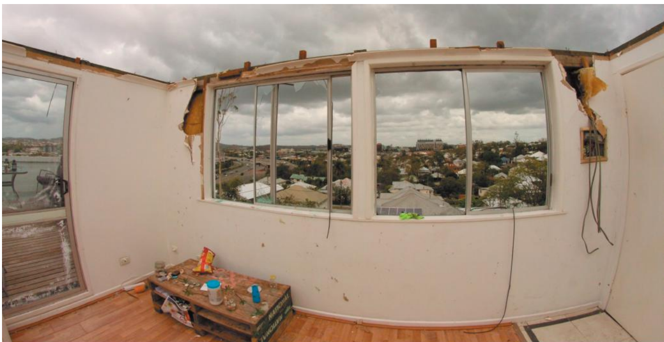
Figure 72: A super cell hit Brisbane on November 28, 2014, causing widespread destruction in a short period of time. In this photo, a roof has been removed from a block of flats. Source: paintings/Shutterstock.
