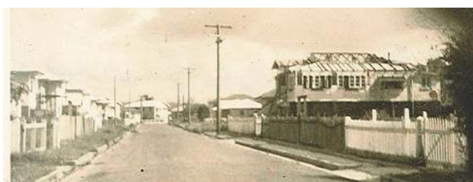
Figure 32: Roof Loss in Norman Street, 1954 Great Gold Coast Cyclone.
