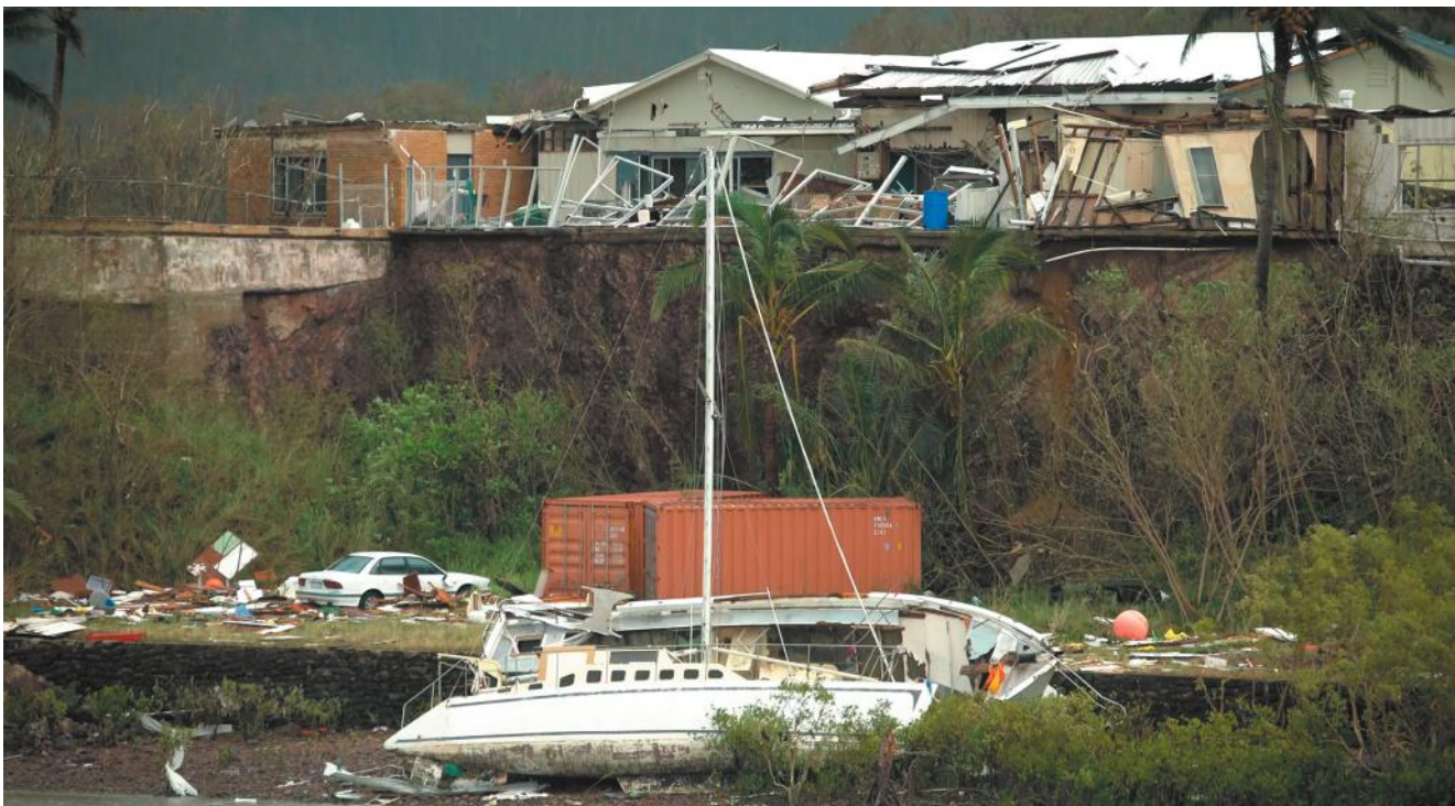
Figure 40: Shute Harbour is littered with debris following Cyclone Debbie. Source: Dan Peled (AAP)
