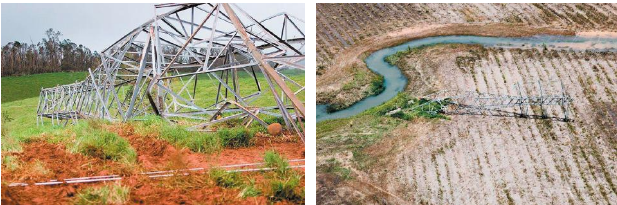
Figure 55: Fallen transmission lines as a result of Cyclone Yasi, 2011. Source: Powerlink
